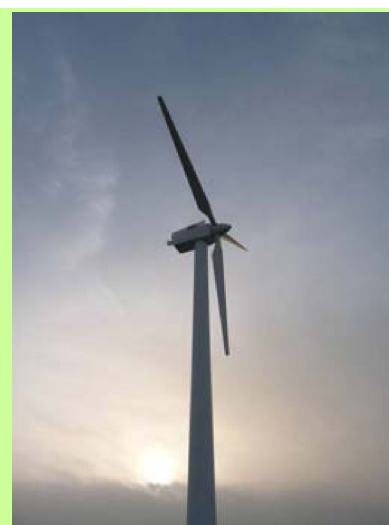
225kW turbine owned and operated by Hockerton Housing Project and visited by 3 groups in the project
